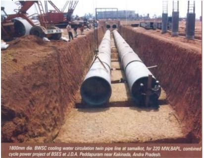
In fact, BWSC pipe is custom designed and an improved version of Steel pipe with lining and outcoating.
