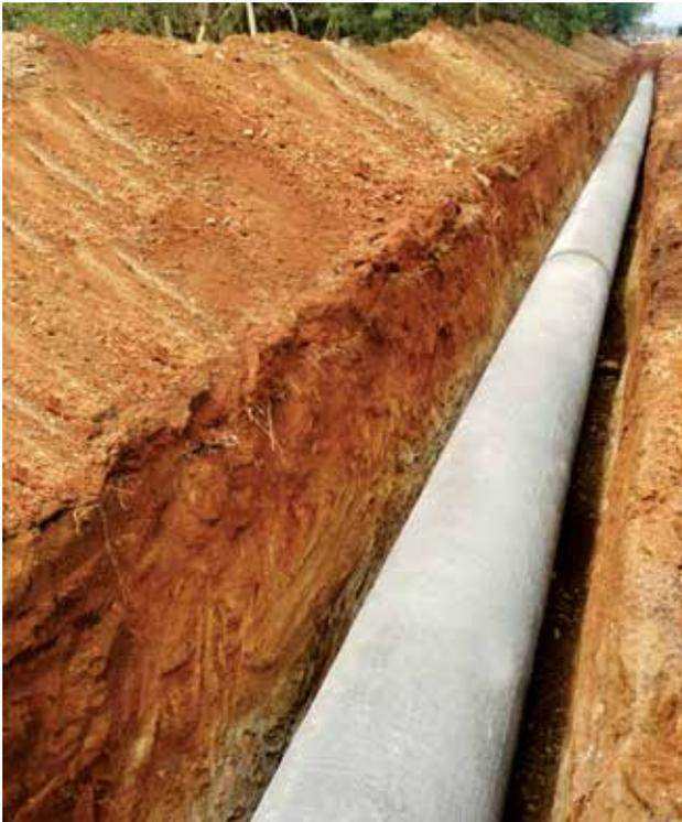
1067 mm dia MS pipeline laying for Madurai Water Supply Scheme, Madurai, in Tamilnadu.
