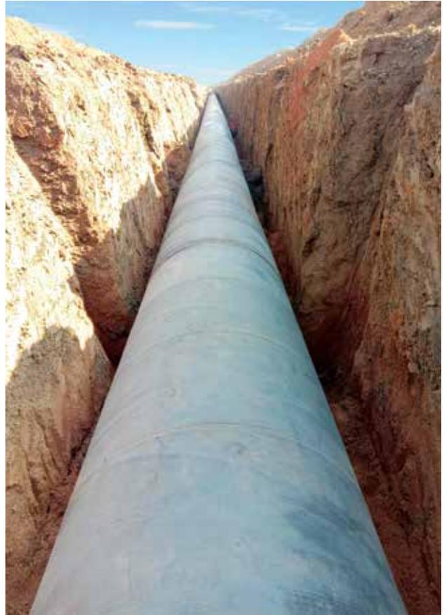
1500 mm dia MS Pipeline laying work for Bilaspur Water Supply Scheme, in Chhattisgarh.
