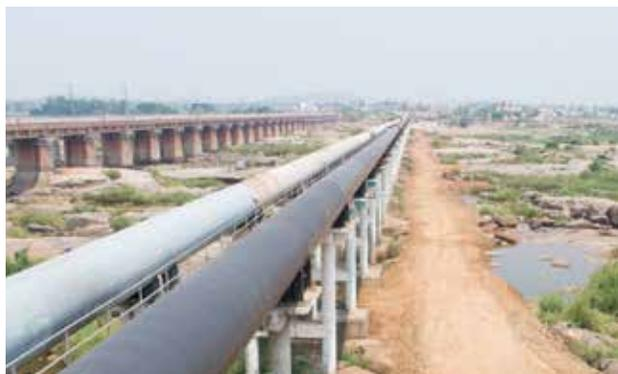
1600 mm dia MS pipeline laying for KPCL Bellary Thermal Power Plant, in Karnataka
