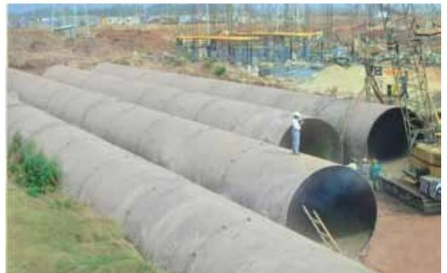
3750 mm dia M.S.pipes with coal-tar coating under erection at D.B. Power plant near Raigarh in Chhattisgarh State for cooling water supply pipe line system.
