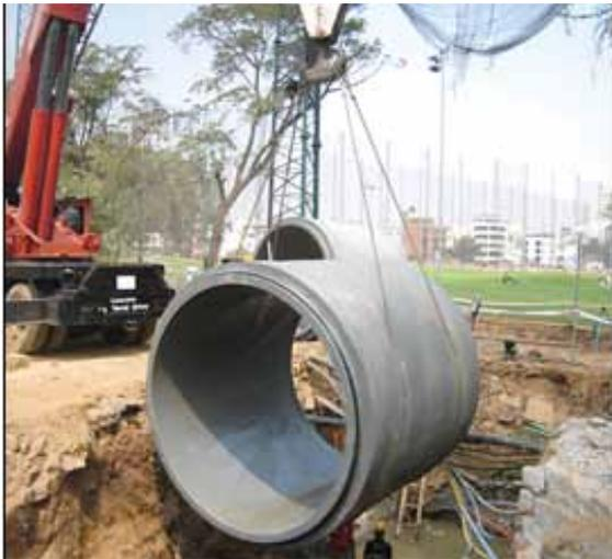
2400mm dia NP3 class RCC pipes for Bangalore Water Supply & Sewerage Board, drainage project.
