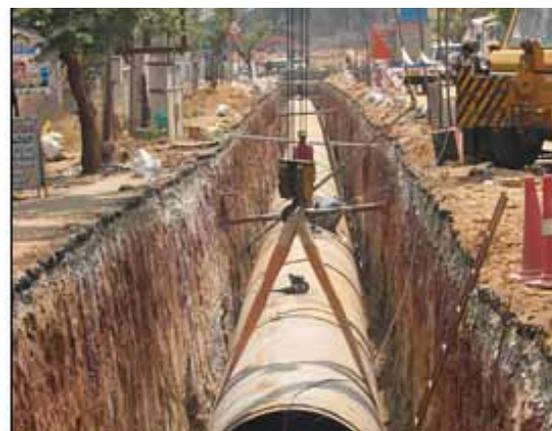
1825 mm dia M.S. Pipes for Cauvery WSS stage IV Phase-II BWSSB W5d Project for drinking water supply to Bangalore
