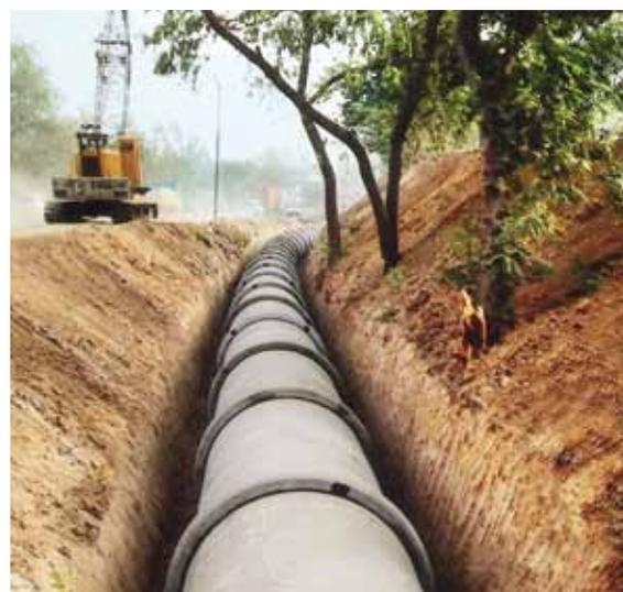
Laying of 2000 mm PSC pipes on concrete cradle bedding at Ghaziabad water supply project
