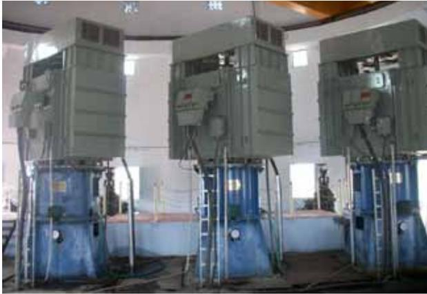
VT Pump & Motors 1000 HP at Dondapadu LIS in A.P
