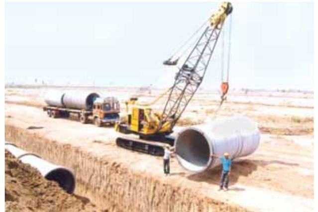
Laying of 2000 mm dia PSC pipes at Pulikanuma Lift Irrigation Scheme in A.P
